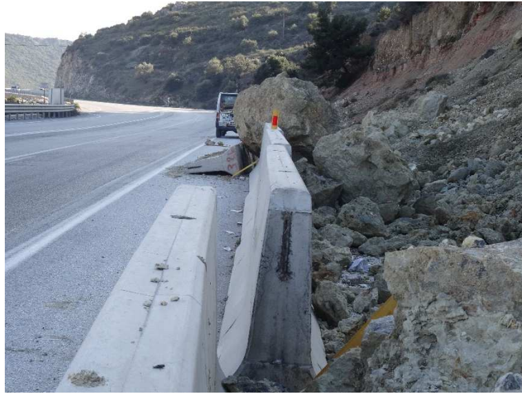
Figure 4. Rockfalls triggered in limestones by 6 th February Kahramanmaraş earthquakes along Hatay – Altınözü highway.
