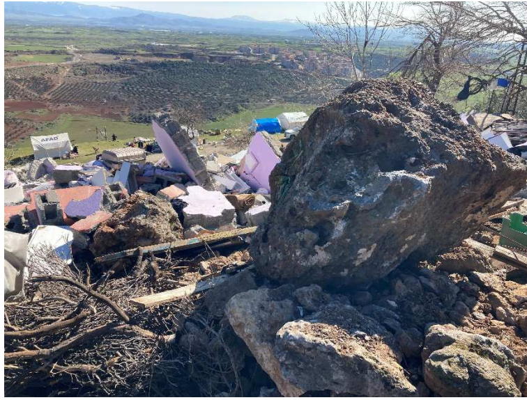
Figure 6. Fallen blocks causing destruction of a residential house in Fevzipaşa-İslahiye district.
